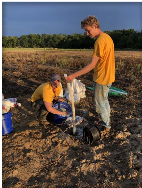
MS students Riley Kniptash and Thomas Doyle backfilling the CMT multilevel.
