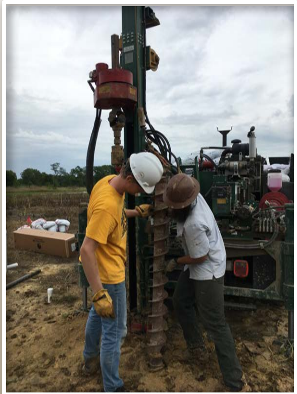
Matthew Streeter (IGS) and MS student Thomas Doyle drilling a borehole using hollow stem augers and the IGS giddings drill rig.
